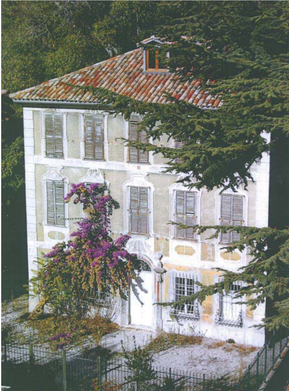
ICRA Net – Villa Ratti before the restructuring's works– Nice (Fr)
